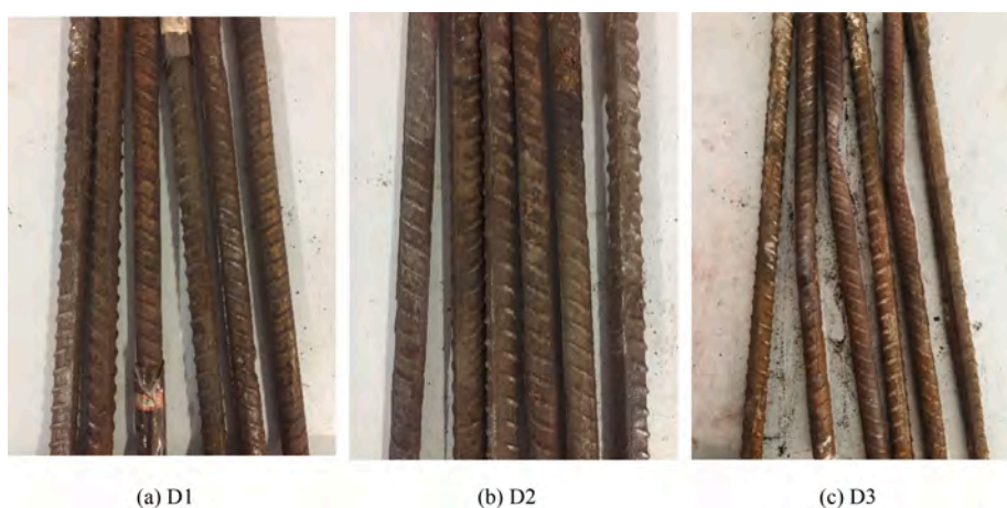
Fig. 7. Images of the concrete reinforcement after varying degrees of corrosion.
